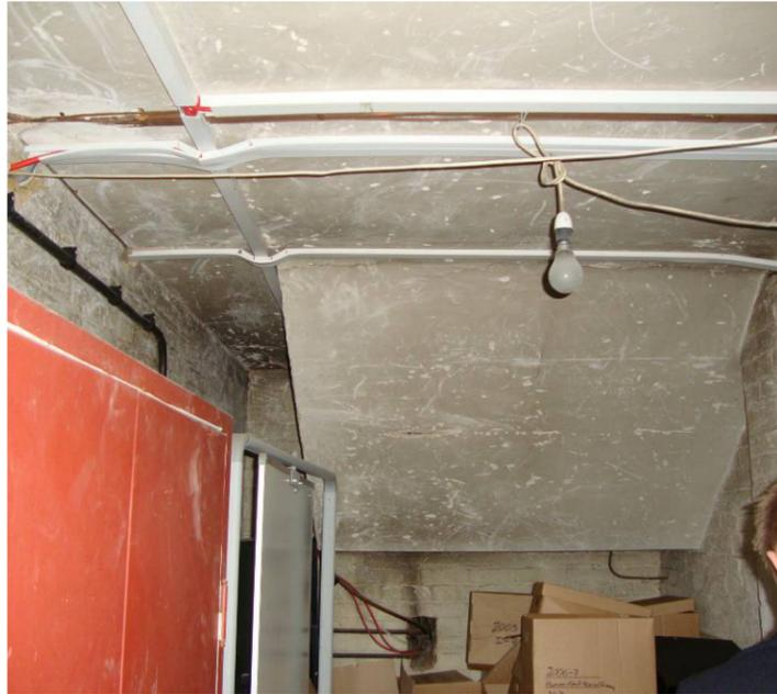
Stair access was required between original lobby level and the ground floor of the southern wing. The concrete stair structure cuts into the loadbearing walls below as shown on the adjacent image. As the lobby level has been raised from its original standing, these stairs have been infilled/framed out but still remain underneath.
