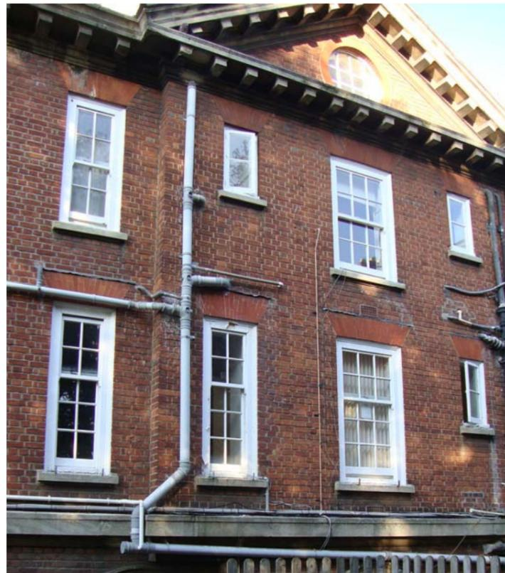
The 1913 Ruskin building was extended to the west in the 1930's using an identical structural form. The extension is keyed directly into the existing masonry facades to form a single homogenous skin.
