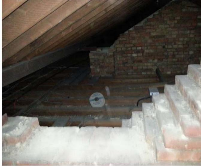
The original Ruskin roof space houses the chimney stacks and provides the location where they traverse from one side of the corridor to the other. These are in good condition.
