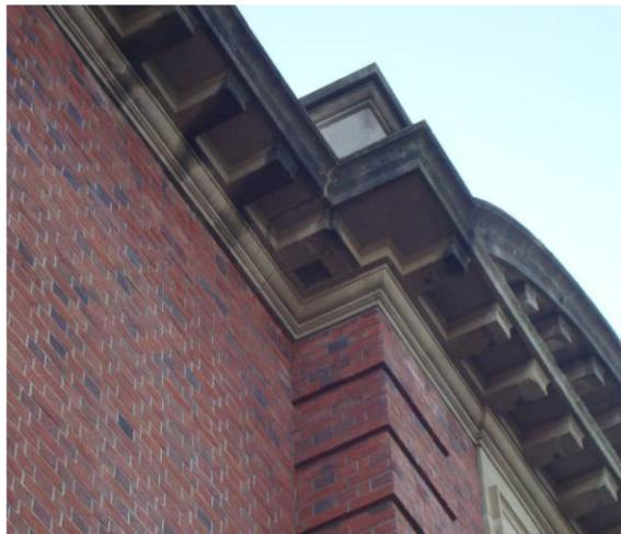
Coping stones running along the perimeter of the building are generally in fair condition although a number are stained due to presence of water within the perimeter gutter that may have leaked or overflowed if blocked.
