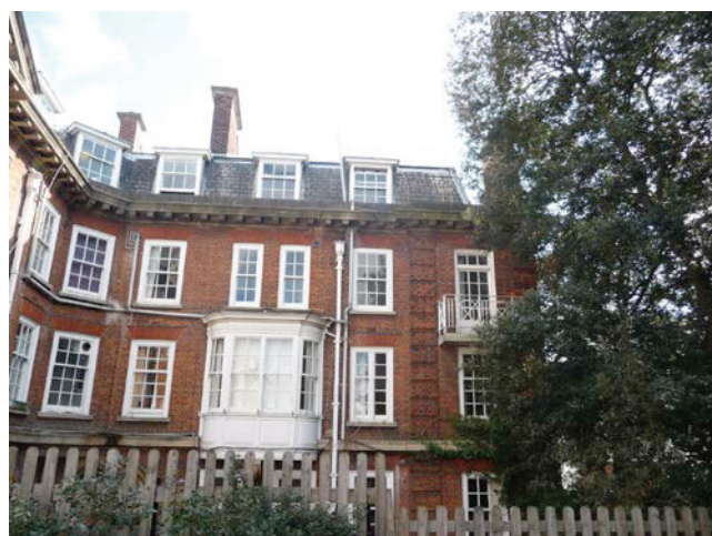
Fig. 1 west elevation, most weaknesses were present in the protective coverings (flashing, tiles etc) found at the curve of the building (Fig. 3).
