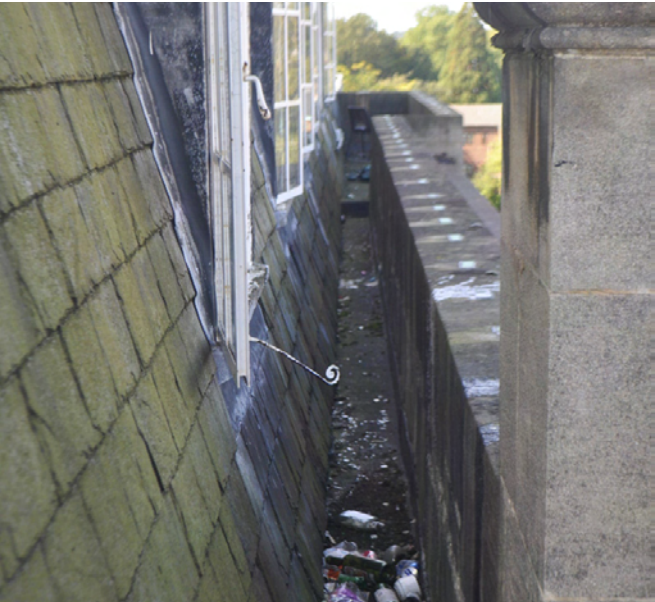
Roof Gutter behind Parapet
