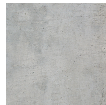
exposed concrete soffits
