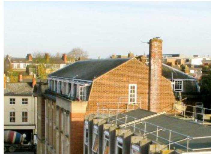
The Ruskin Building - Existing Mansard Roof
