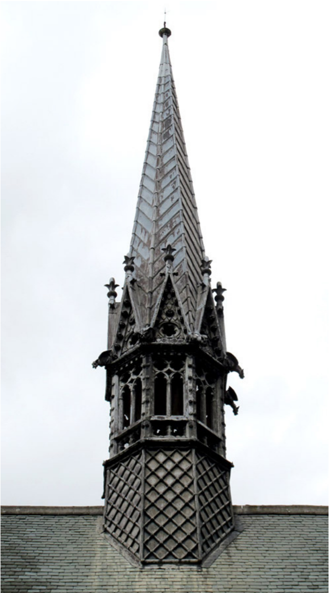
Lead lattice work to the lead fleche on Exeter College Chapel
