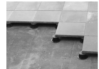
Pedestal Paving System
