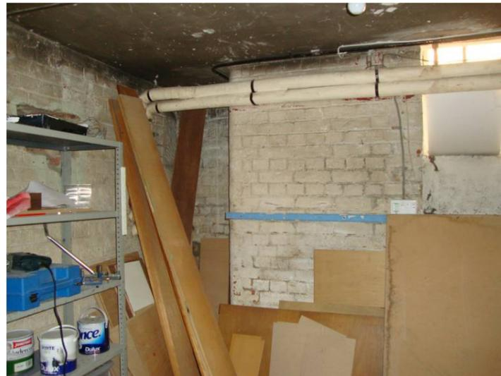
Basement retaining walls are formed in loadbearing masonry. They appear to be in reasonable condition.
