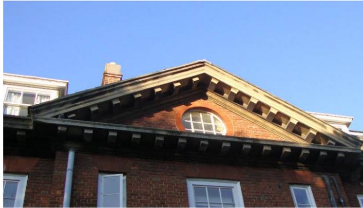
Three stone pediments feature on the building. The stonework generally appears to be in good condition. The very edges of the pediments (directly adjacent to perimeter coping) are subject to the similar staining as the perimeter coping.
