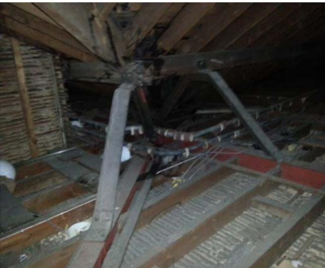
The roof structure is formed from timber rafters picked up on triangular steel frames located either side of the corridor walls, the structure appears to be in good condition overall.
